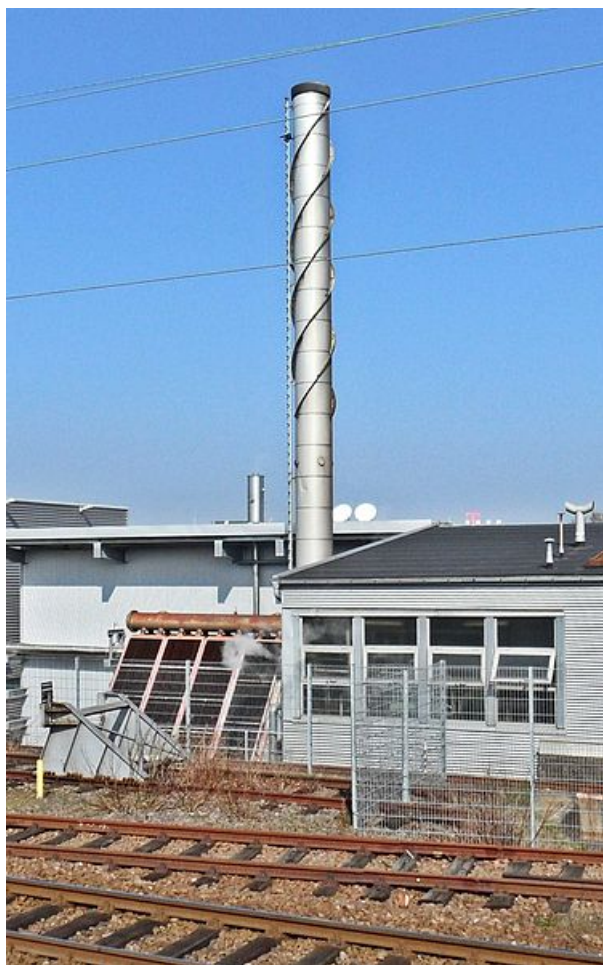
Figure 7.3: Chimney with helical strake
